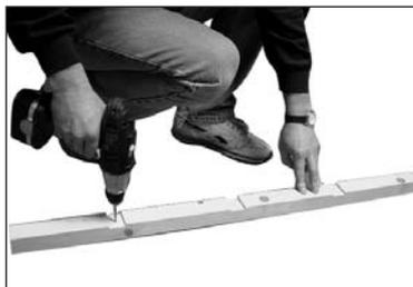
1 Drill through the centre of each notched area on both posts where a 'step' will be screwed into place.
