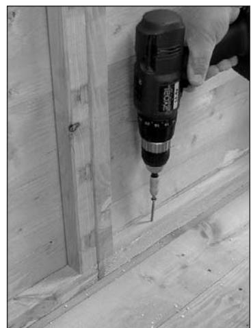
4 Drill and screw all side panels to the floor on the inside of the building using 1x 60 mm screw per panel, into a floor joist if possible.
