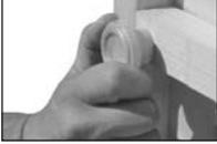
4 Place the three false hinges in position on the front of the door, ensure the screws go through the framework on the back of the door. Screw into position using 4x 25mm black screws per hinge.
