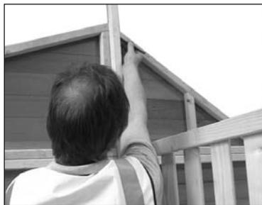
4 Place the balustrade railing against the side of the upstairs floor and against the gable wall. Mark on both sides of the balustrade railing where the railing (A3) meets the bottom edge of the gable framework. Connect the two marks and cut the balustrade railing.
