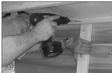
3 Fix the upstairs floor to the framework of the two side walls using 2x 80 mm screws.
