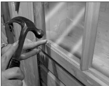
3 Hold into position with four pieces of beading (B4). The beading may need to be swapped around to get the best fit. When satisfied secure into position using 2x 15mm panel pins per piece of beading.
