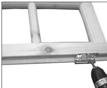
3 Place the hinge back onto the insert and screw the inner piece into position using the predrilled holes in the hinge and 2x 25 mm screws. Repeat.
