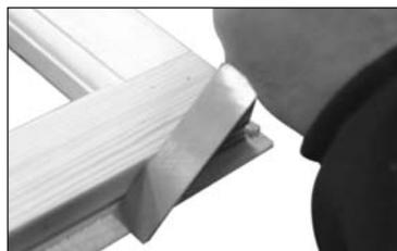
2 The hinges should be recessed into the window frames (B2) to a depth of 3mm. To do this: place one hinge on the inner rebated part of the top of the window. The rounded part of the hinge should sit above the outer edge. Mark the position of the hinge on the weather proofing part of the window insert. Remove the hinge. Chisel out the timber to a depth of 3mm in the positions marked. Repeat.
