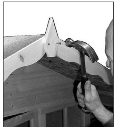
3 Fit fascia and diamond to front and back roof edging. The profiled fascia (J1) goes at the front of the building. Secure using 3x 40 mm nails for each length of fascia and 2x 40 mm nails for each diamond (K).
