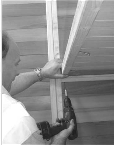
2 Attach the floor in position using 2x 60 mm screws at each side, up through each bar and into the floor.
