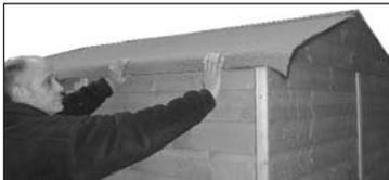
2 Measure out and cut at 2000mm x 3 strips. Lay one piece of felt along the longest lowest edge of the roof. An overhang of approx 40mm should be allowed on each of the 3 sides. Secure using 13 mm felt nails at approximately 100 mm intervals, but do not nail down along the centre of the building.
