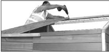
1 Attach a piece of framework (H1) to one edge of one large roof piece (H) using 4x 25mm screws. Place this roof panel in position at the rear of the building. Ensure that the roof is flush with the back wall and point of gable. Screw into place using 3 x 25mm screws into the back wall and 2 x 25mm screws in each roof bearer (H3). Repeat for other side.
