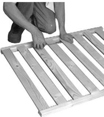
2 Space out remaining slats (at approx 60 mm intervals). Drill and secure in place using 2x 25 mm screws per slat, one at either end.
