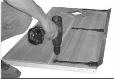
5 Fit the door to the panel using 25 mm screws in 10 of the available holes spaced evenly along the length.
