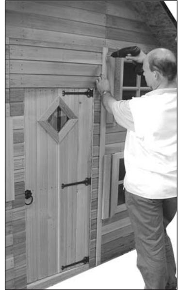
2 Fit coverstrips (G) over each panel joint and in each corner, using 3x 40 mm nails per piece. There are two small coverstrips to cover over the gable joints. Secure using 2x 40 mm nails per piece.
