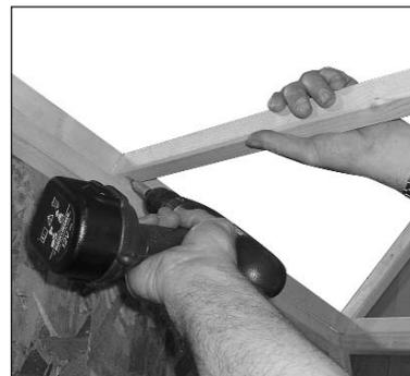
9 Attach the framework of the balustrade railing to the roof bearer using 1x 60 mm screw, placed at an angle.
