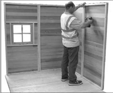
2 The double window (BB) panel must go at either side of the front. Decide where you would like the window panels. Place 2 wall panels (D) in position in a back corner. Drill guide holes in one panel only. Screw to the other panel using 2x 60 mm screws in each panel. Repeat.
