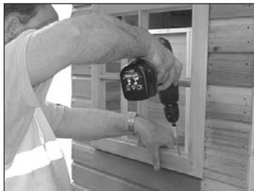
1 Fixed windows (2 as standard) – one of which MUST be the top window. Drill guide holes, 2 at the top of the frame and 2 at the bottom. Secure in place using 4x 60 mm screws
