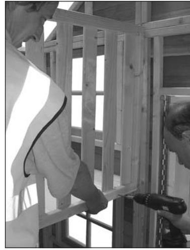
6 Place the balustrade railing in front of the upstairs floor, flush to the front wall. Note: slats face the upstairs. Drill and screw into position using 3x 60 mm screws along the bottom of the balustrade into the upstairs floor.
