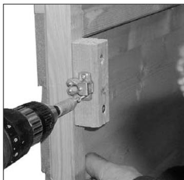
3 Close the door and attach the door catch together and mark the required position of the door catch housing. Secure using 2x 25mm screws.
