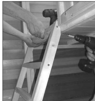
8 Attach the ladder (A4) to the upstairs floor using 2x 60 mm screws.
