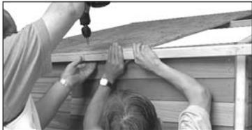
2 Attach a further roof piece (H) and a further piece of edging framework (H1). Attach using 3x 25mm screws in each bearer and 2x 25mm screws into each roof edging piece.
