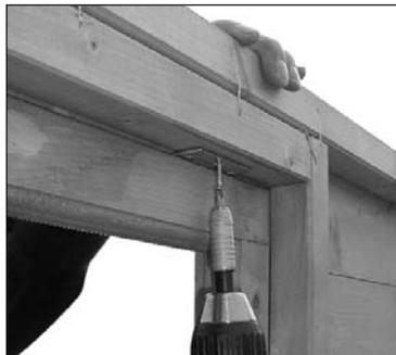
4 Place the window into the aperture. Secure the window to the panel using 3x 25mm screws per hinge, again through the predrilled holes in the hinge. Repeat.
