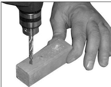
1 Drill x 2 holes into the wood block and secure to inside of door opening flush with the aperture using 2x 60mm screws.
