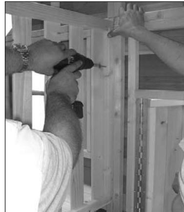
7 Attach to the front wall using 2x 60 mm screws.
