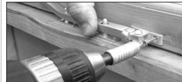
7 Fit the Casement Stay on the window using 2x 25mm screws.
