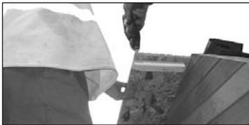
4 Fit 2 small roof blocks (H3) to centre of overhang and 1 block half way along each half roof. Secure in position using 2x 25mm screws per piece.
