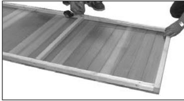
1 Place a bar in one plain side panel (D). Measure from the bottom of top piece of framework of the panel to the top of the bar 740 mm. Drill the edge of the panel and screw the bar into place using 1x 60 mm screw at either end. This panel MUST be fitted opposite the double window panel.
