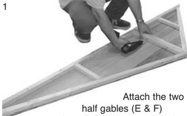
1 Attach the two half gables (E & F) together. Drill and screw fix using 2x 60 mm screws. Repeat.
