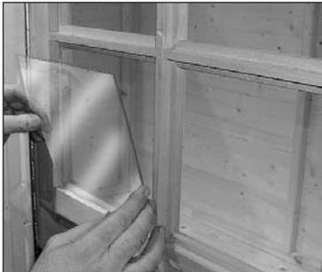
2 Place glazing material (B3) into the aperture of each window.
