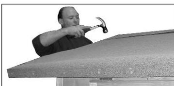
4 Place the final strip over the ridge overlapping the other 2 pieces already laid. Secure using 13 mm felt nails as previously.
