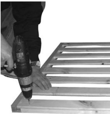
3 Place the 630 mm framework behind the edge of the slats. Drill and screw into place using 3x 25 mm screws through the slat into the framework.
