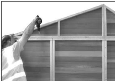
3 Secure the gable sections using the pre-drilled holes. Screw through the wall into gable. 4x 60mm screws. Repeat.
