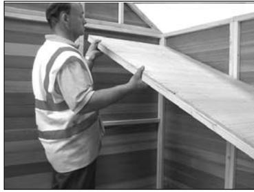
1 Place the upstairs floor (A1) on top of the bottom window and the bar previously fixed to a plain side panel.
