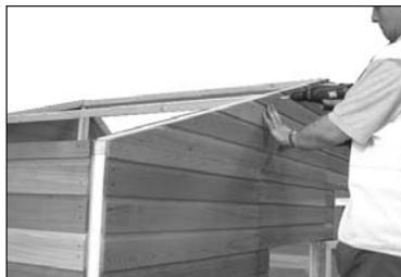
5 Using the predrilled holes in the gables, fit four roof (H2) bearers using 8x 80 mm screws. One in each end.
