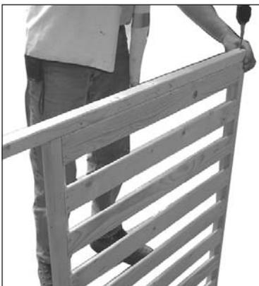
4 To the other end fit the 1300 mm (A3) piece of framework. The piece of framework should be fitted flush with the slats. Drill and screw into place using 2x 60 mm screws, one at either end.
