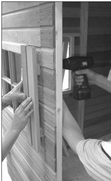
1 Fit shutters (B1). One person to hold in place and another to secure from the inside using 4x 25 mm screws, 2 into each block.
